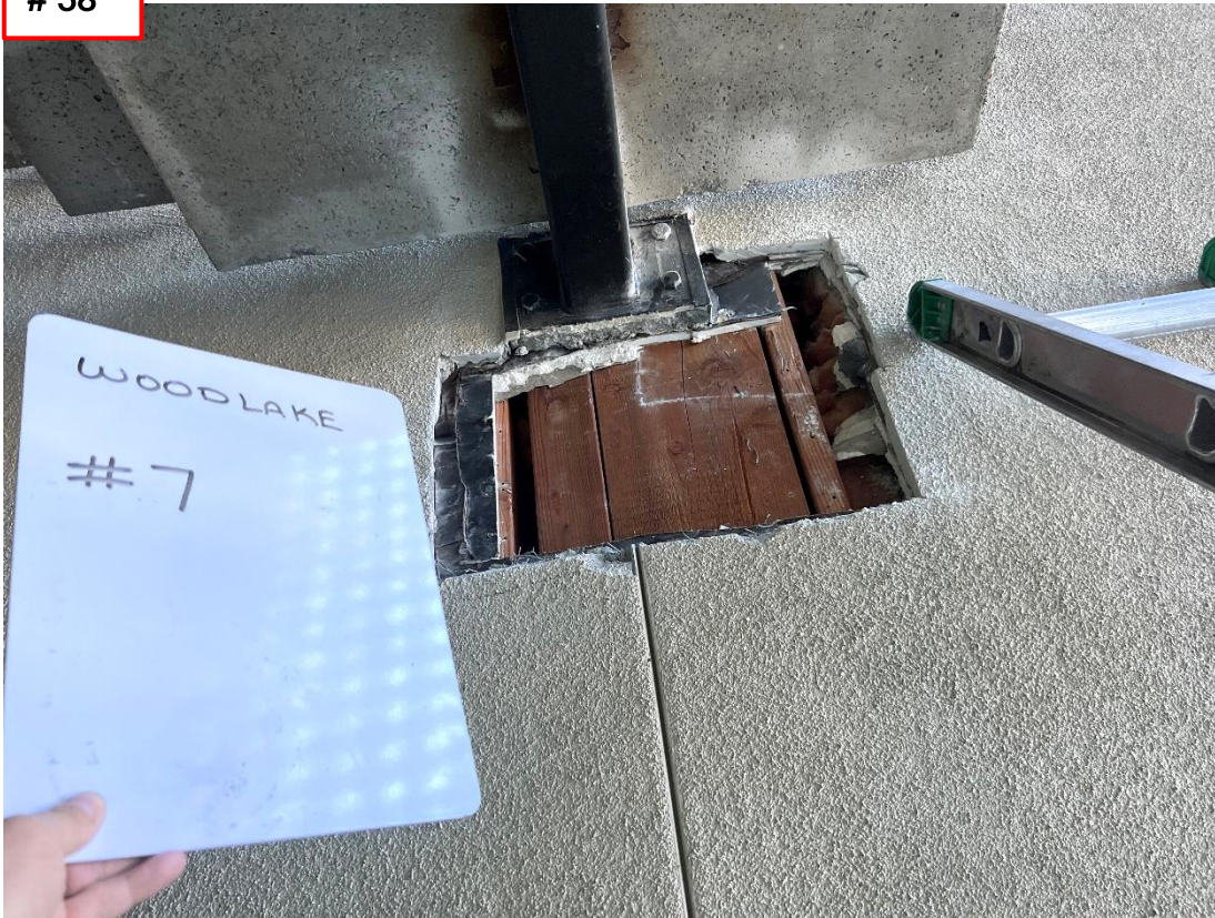
Location # 7 Staircase attachment to wall
