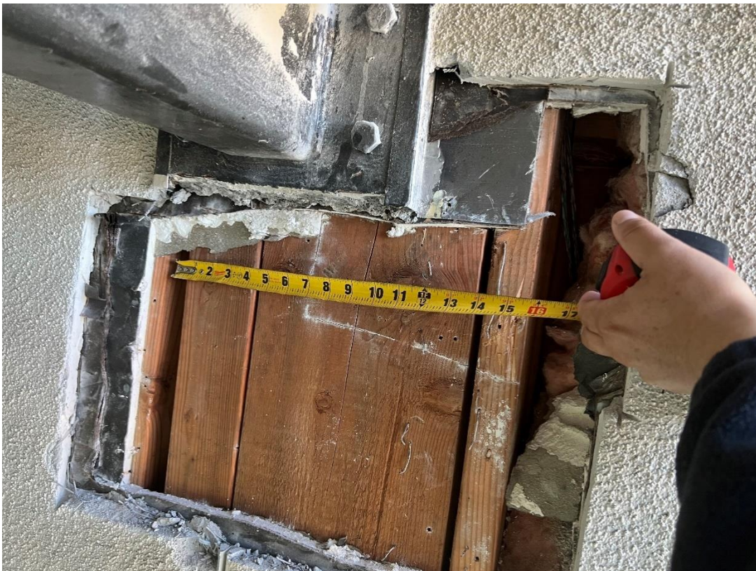
Location # 7 Staircase attachment to wall - no damage to framing
